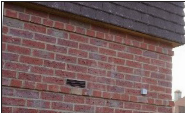
Projecting horizontal perpendicular courses, tile-hung first floor
