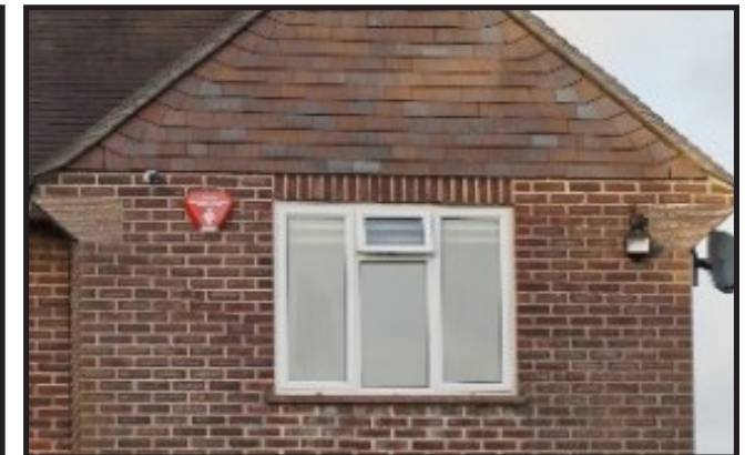
Tile corbelling to hung tile gable end
