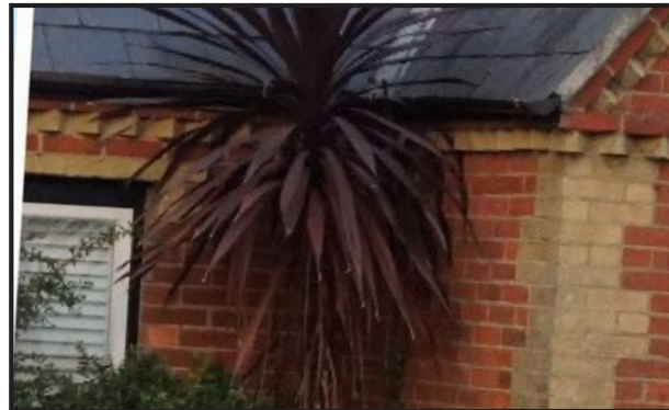
Diagonal brick course to eaves and gable with colour contrast
