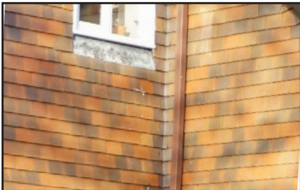
Castellated projecting brick course trim to hung tiles
