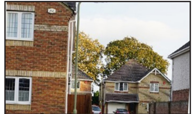
Colour-contrast brick coursing reversed behind, projecting box course supporting white contrast first floor on right.
