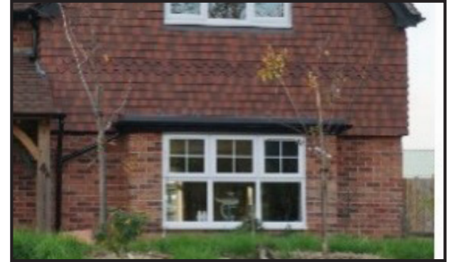
Brick ground floor with pattern and coursing of hung-tile first floor and gable
