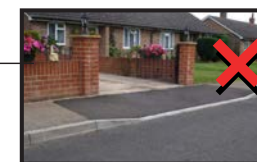
Interrupted pavements over driveways
