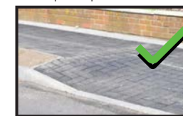
Uninterrupted pavements over driveways
