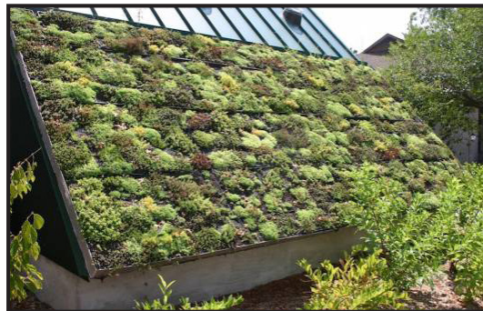
Orientate green roofs and walls to optimal sunlight radiation and minimise the effect of overshadowing
