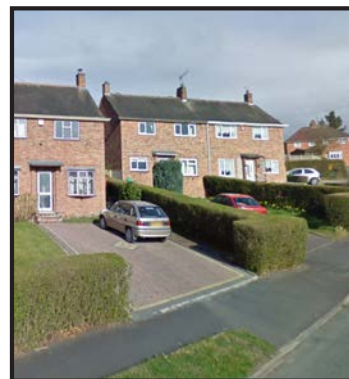
Stanley Rd. On-plot parking on driveway
