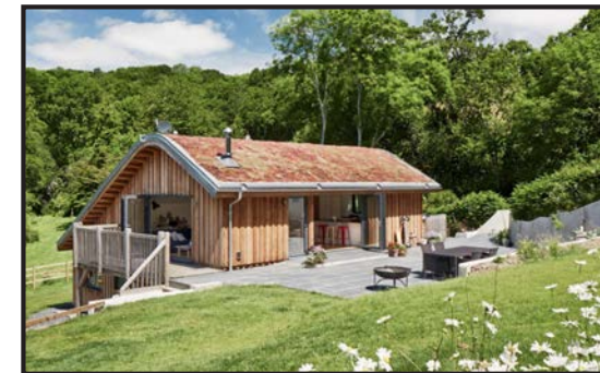
Protect green roofs and walls from excessive wind levels, in this case the sloping site assists in the protection of the roof
