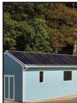
Often, covering a whole side of a roof is the best way to relate to its general shape
