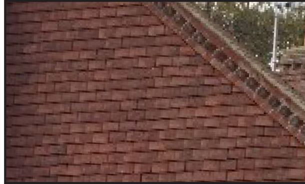
Diagonal brick course in corbel to chimney, roof and hung tiles
